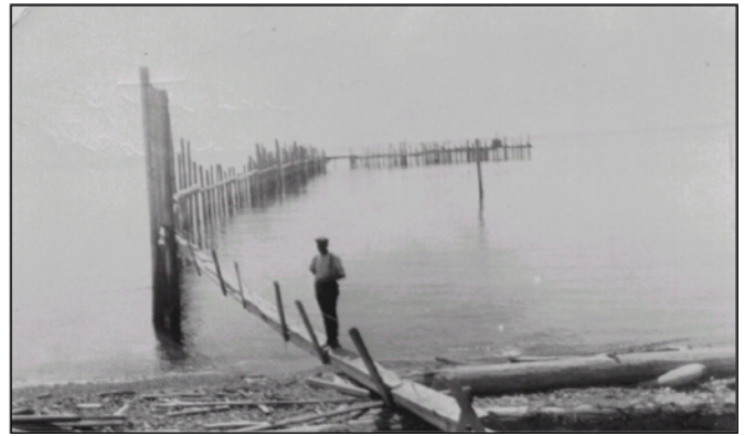
The lead to the fish trap on Johns Island tied into the shore to direct fish into the trap.
