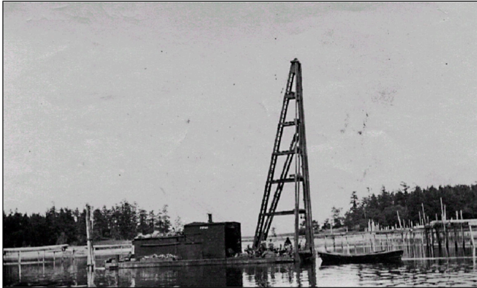
Driving pilings for the fish trap off the southeast shore of Johns Island. Shallow water at Johns allowed fixed traps to be used rather than floating ones.
